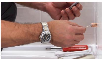
**7.** Then apply epoxy completely to inside of tube in wall.
