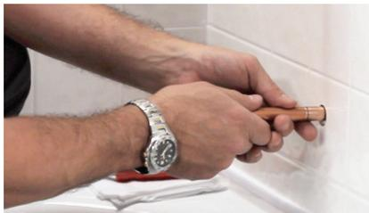
**4.** Dry fit repair adapter to make sure it fully slips into copper tube in wall.
