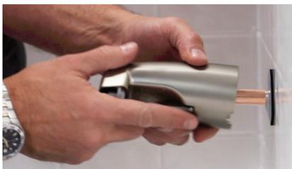
4. Remove backing strip on Dry Seal Pipe Collar. Push Dry Seal Pipe Collar over tube and apply firmly to wall. Push the SmartSpout onto the tube, and against the wall.
