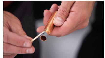
**6.** Working quickly, apply epoxy completely to outside of reduced end of repair adapter.
