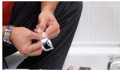
**5.** Squeeze one side of epoxy pouch to burst the middle seal. Work epoxy to other side and mix thoroughly until gray color appears.
